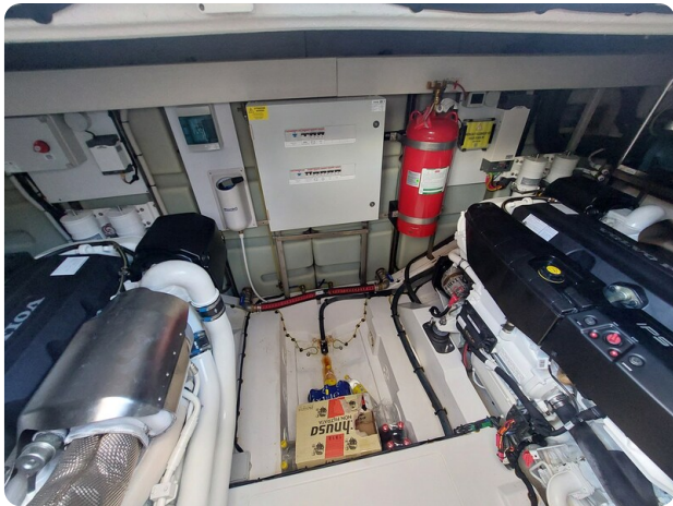
Azimut 53 Fly engine room
