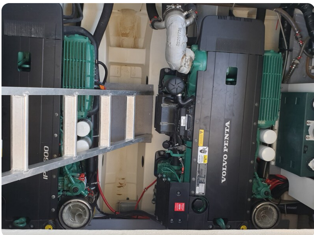
Beneteau MC5 engine room
