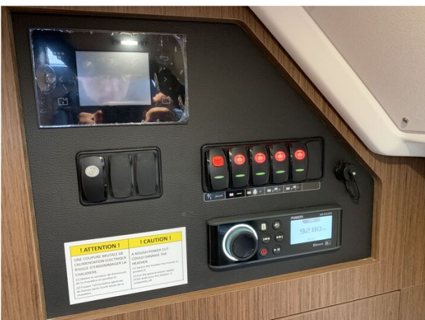
Jeanneau NC 37 twin diesel cruiser - audio controls and switch panel
