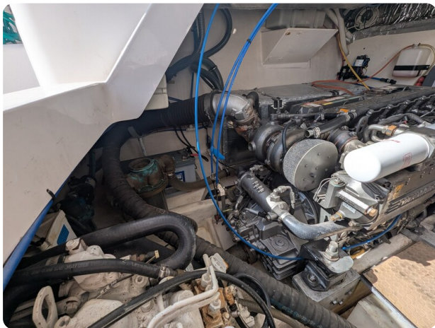
Luhrs 36 Open engine room detail
