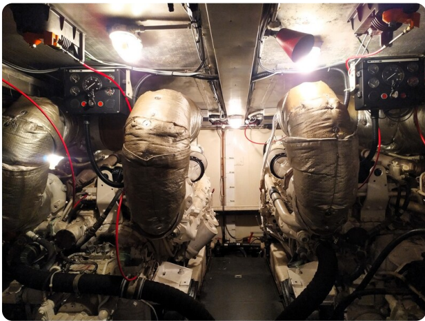
SANLORENZO SL 62 Engine Room
